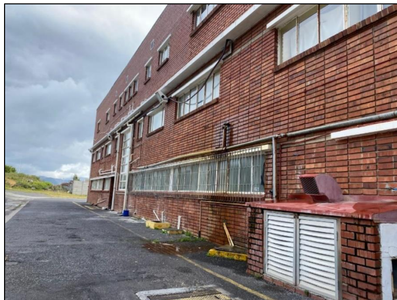
Figure 7. All outdoor waste bins have been removed and secured at Job Maseko.
